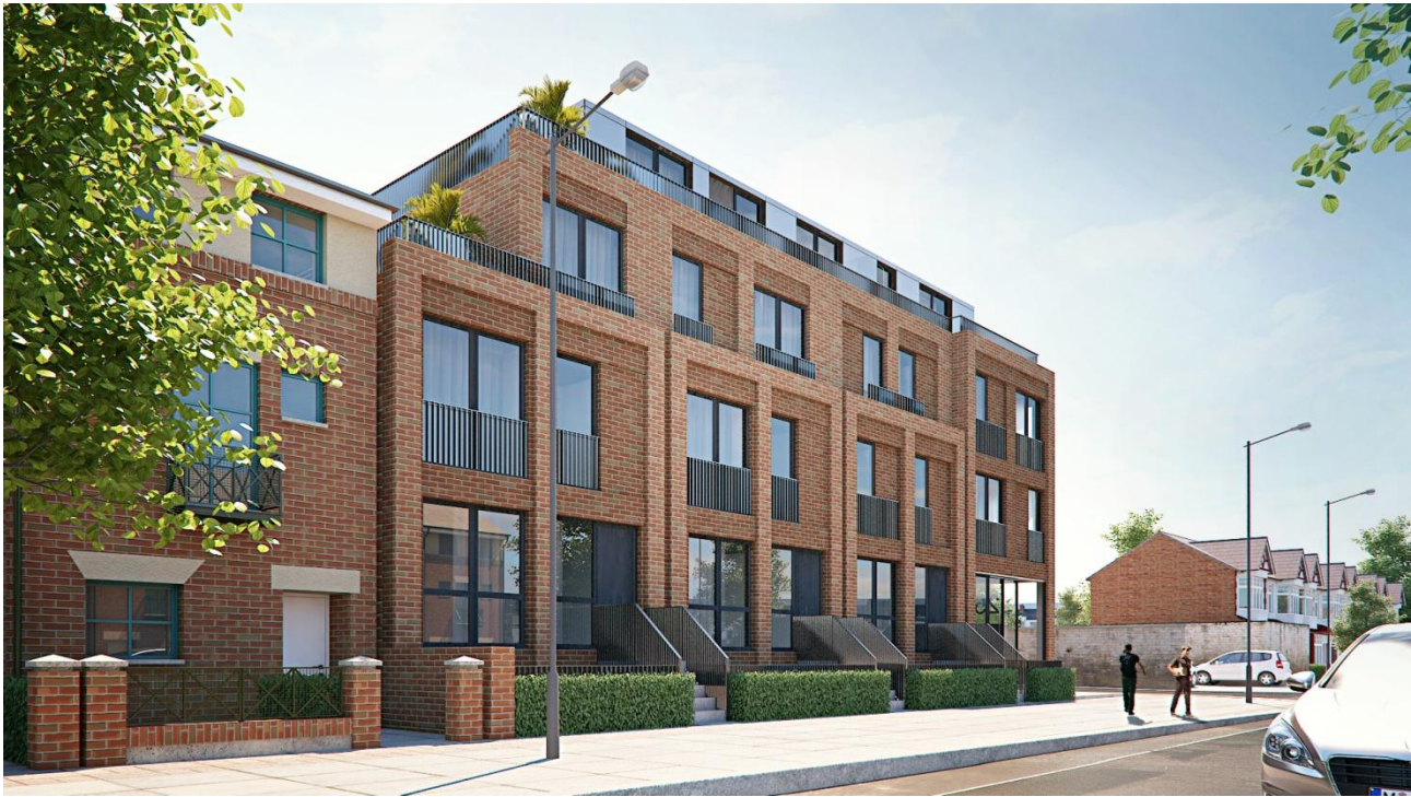
Visual along Lordship Lane looking west
